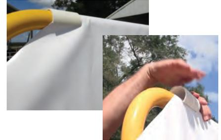
13. Secure the curtains to the top rails and the vertical posts with PVC clips. Use 3 clips each on top, front and rear rails. Get them started by hand and use the rubber mallet to fully set or a big smack with your hand. If not present drill 8 5/16" holes thru the vinyl using the holes on the top rail as a guide.
